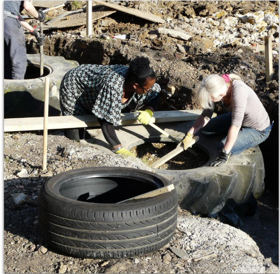
Community building at Tulsa Hill by Richard Dormandy (2017)
